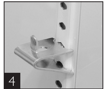
4 Shelf clip installation complete
