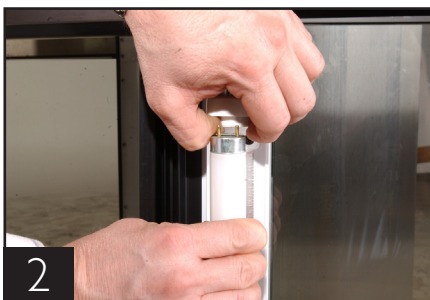
The lamp holders are spring activated. Pull the top lamp holder up and push the bulb down at the same time. This will leave enough clearance to remove the bulb.
